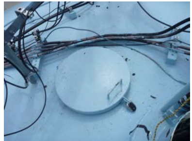
Interior Wet Hatch (Roof)
